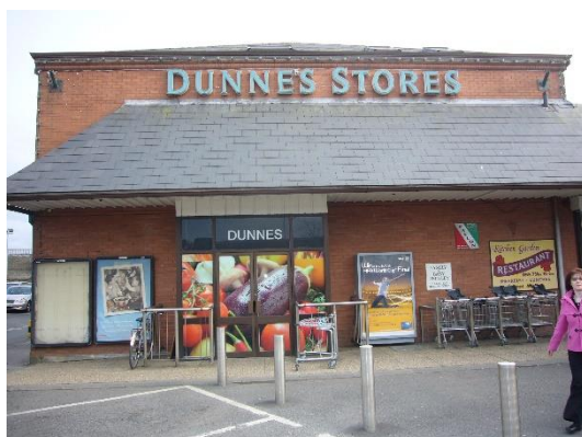
Entrance to unit
